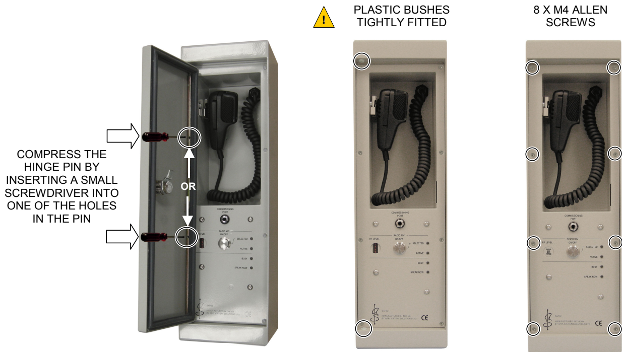
Figure 23 SAP02 Door and Front Panel Fixing
